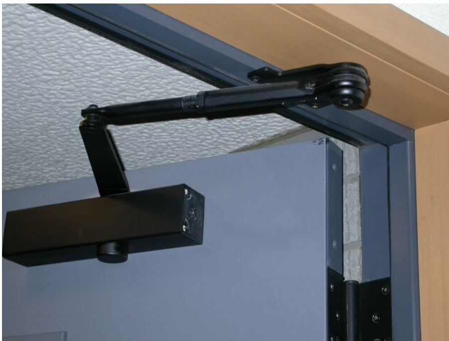
Figure 3.2: A good door closer should close automatically, close in a gentle manner and close as fast as possible.
