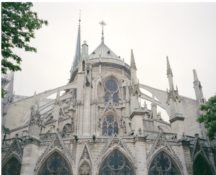
Figure 7: Structural Design: Materials technology is littered with equations, etc that then feeds into structural design. Flying buttresses were designed to balance these equations and hence the building itself.
