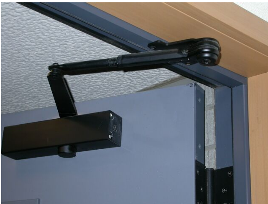
Figure 1: A good door closer should close automatically, close in a gentle manner and close as fast as possible.
