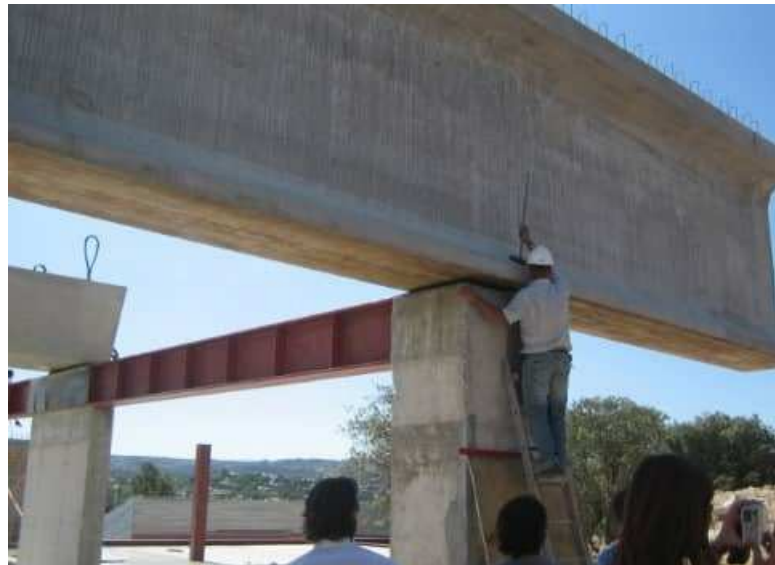
Figure 2.14: For simply supported beams, there is nothing keeping the beam 'straight' at the supports... the bending moment M is zero at the ends. Of course, the deflection y is zero at the ends.
